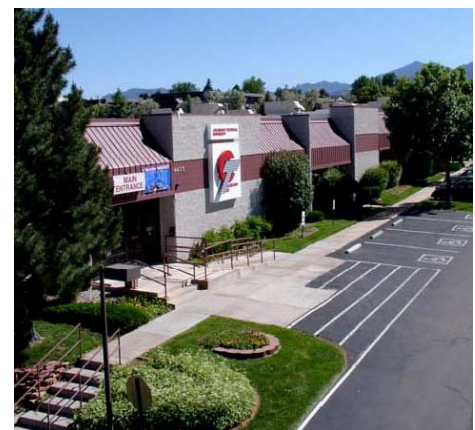
A sub-meter that measured landscaping water was installed at the above 121,000 sf property resulted in an 88% reduction in annual wastewater billing.
